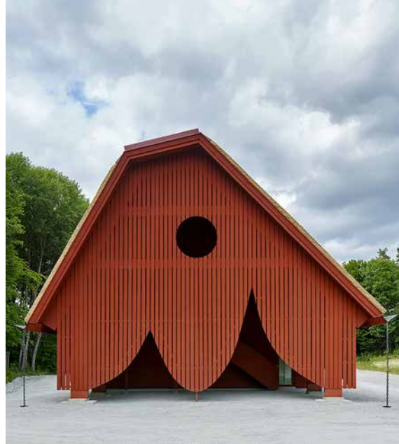
ERIKSBERG ENTRANCE BUILDING, SWEDEN ARCHITECT: SANDELLSANDBERG · PHOTO: ÅKE ESON LINDMAN
