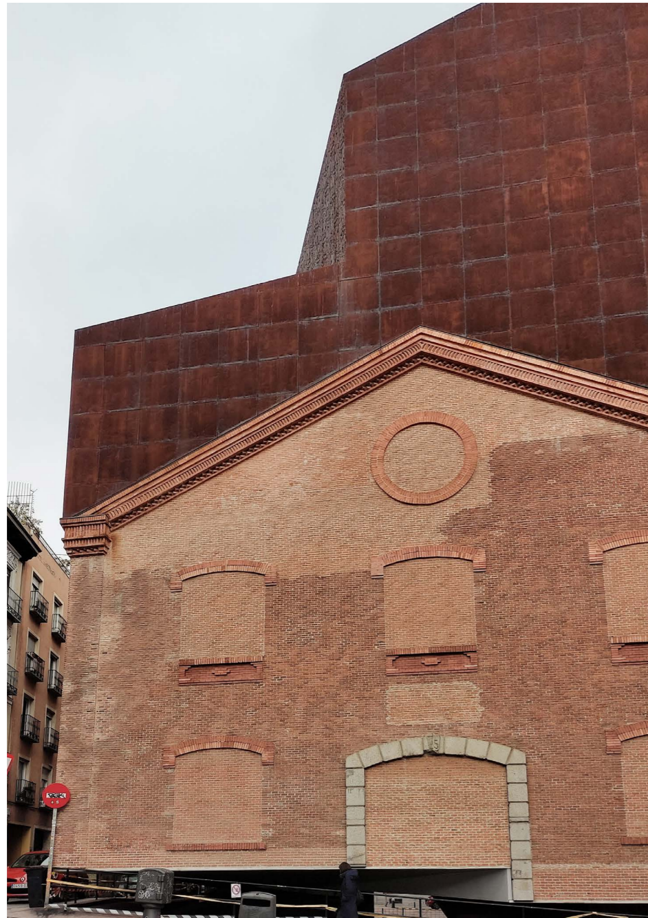
The facade seems to hover over the ground, playing with the heaviness of the bricks and the illusion of weightlessness. The metal panels allude to the industrial background of the building, while the shape provides a very modern touch.
