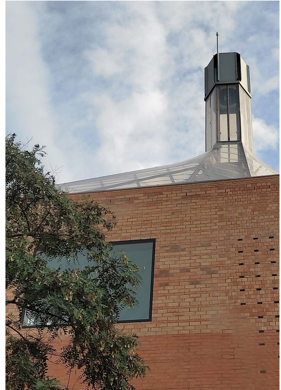
The air inside the solar chimney is heated by the sun and rises, resulting in a draft that moves hot air from the building without the use of energy-costing systems.
