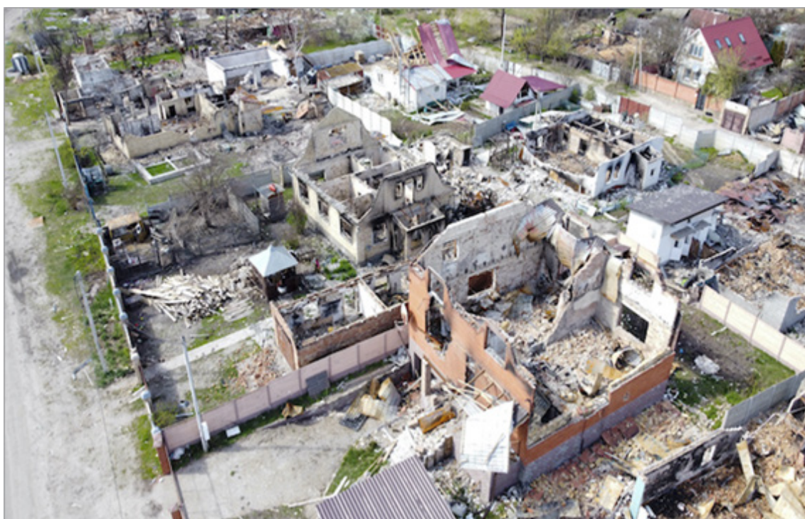
Fig. 4. Air view of the destruction in Lisova st, Moschun. Photo credit: Olena Oliynyk 2022.
