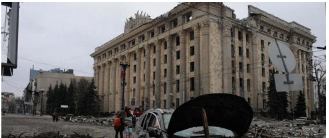
Fig. 9. The administrative building destroyed in Kharkiv. Photo by Oleksandr Bouryak 2022.
