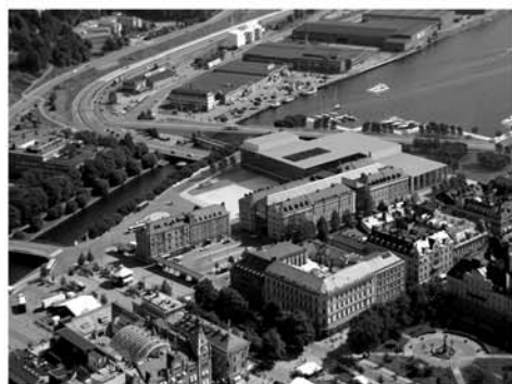
Indoor Communication Aerial View
